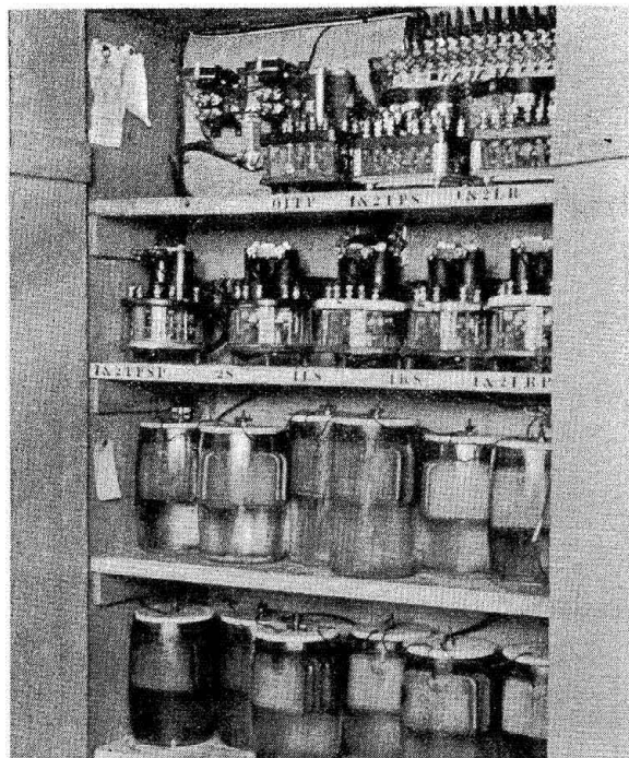
Relays and battery in station at Beloit
