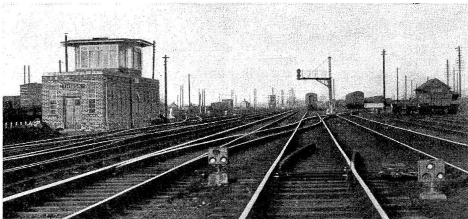
View of Thirsk interlocking, showing, in the foreground, the position-white-light shunting signals
