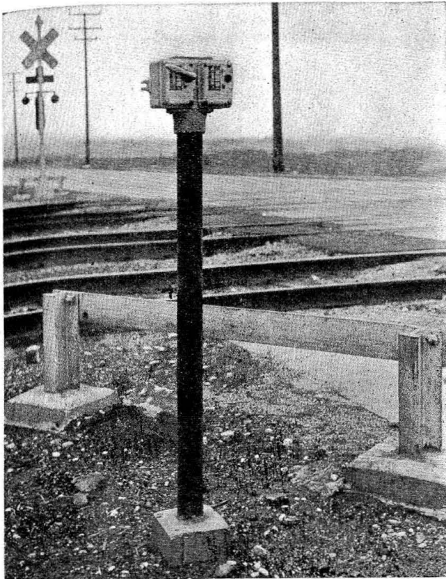
Control station in which a four-way switch is used. . . . The unit at the right, on the top of the pipe stand, is the momentary-contact special-control switch (lever has been removed) which, if in service, would enable the foreman of a switching crew to stop the operation of the flashing-lights when the track circuit is occupied. This momentary-contact switch has been tried out but is not now in service; it may be used in the future, however, if appreciable delays to highway traffic are encountered due to trains standing on the track circuit but not actually on the crossing
