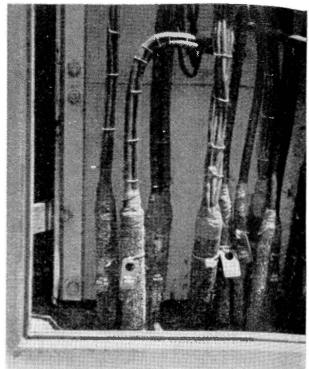
View of cable entrance compartment in end of instrument house
