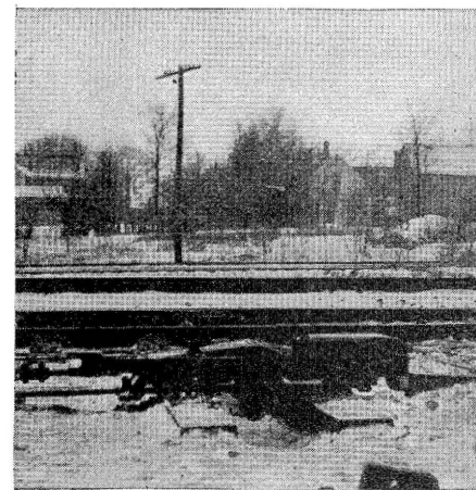
Spring switch with facing-point lock on the Great Northern
