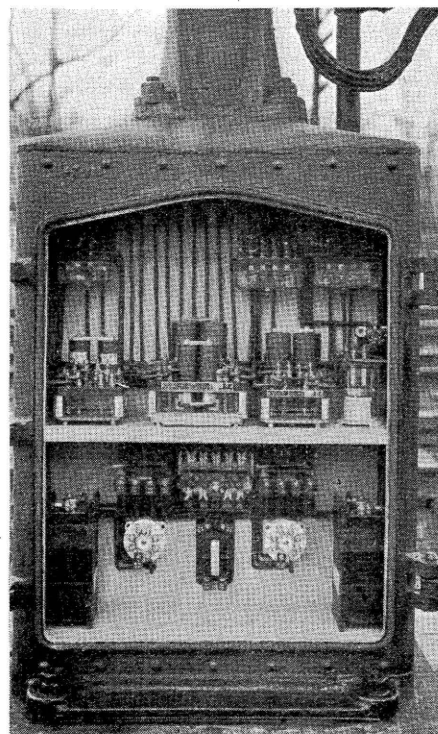
Track batteries are located in lower shelf
