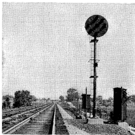
One of the new automatic block locations using position-light signals
