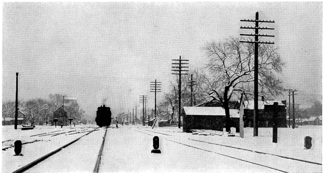
Eastbound Union Pacific train passing over the crossing—Note the three color-light dwarfs in the foreground
