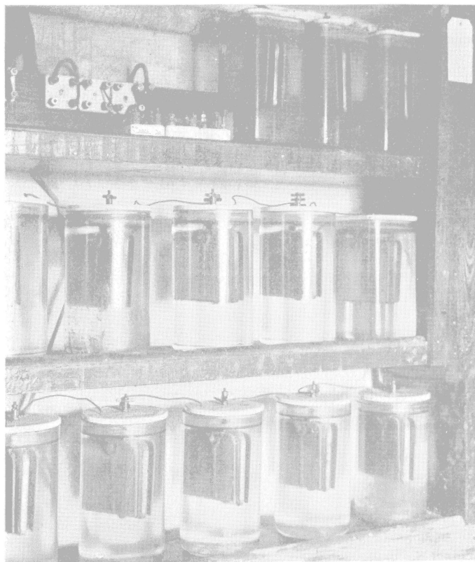
The control and operating circuits are fed from primary battery
