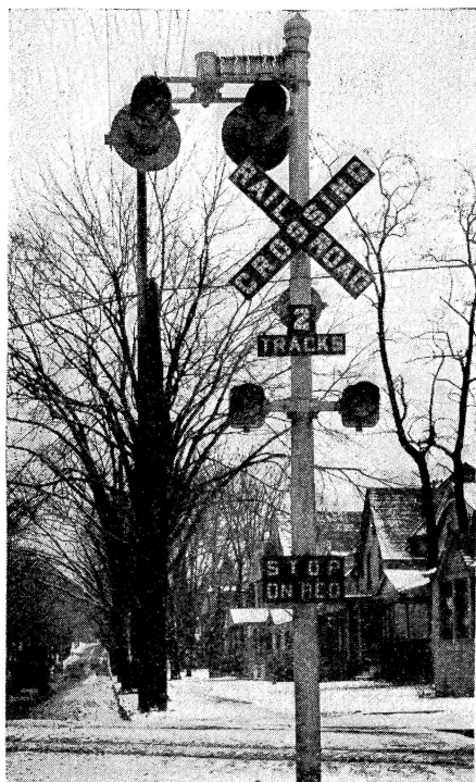
Cantilever mounting for extra flashers at West Main Street, Kalamazoo, Mich.
