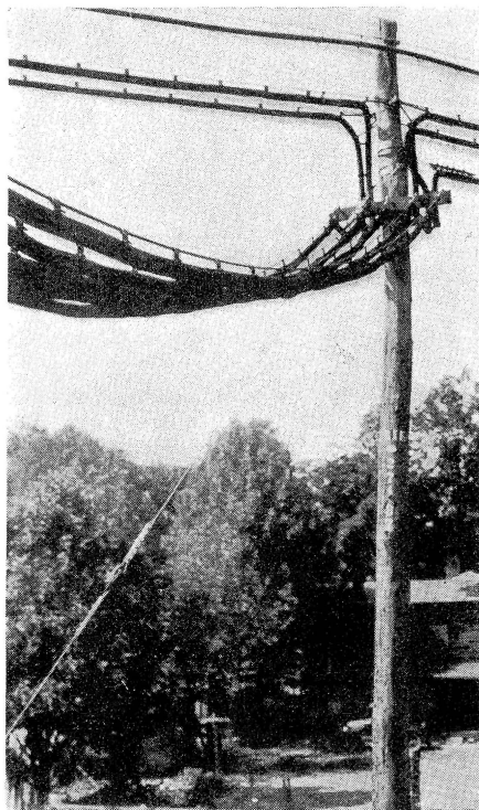
Cable lead from pole to instrument house at Southport Junction
