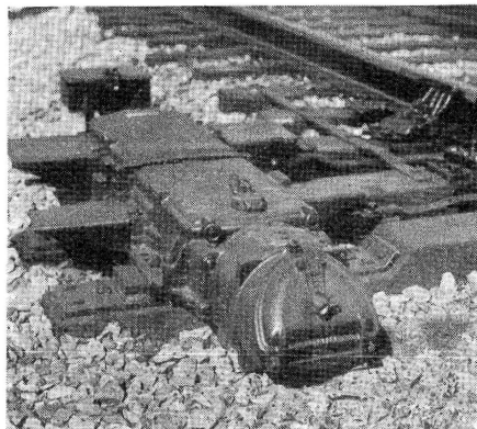
The ties are dapped so as to lower the switch machine with reference to the rail
