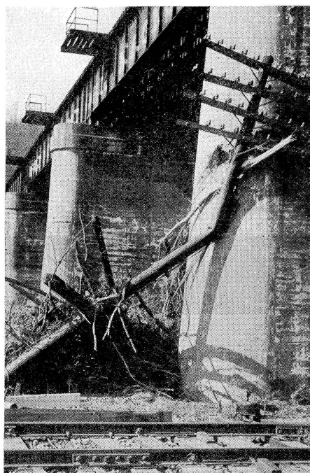
On the B. & O. the force of the flooded streams broke poles to pieces
