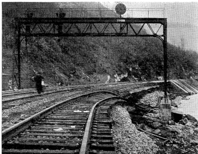
Signal bridge foundation and No. 3 main line undercut near Johnstown, Pa.
