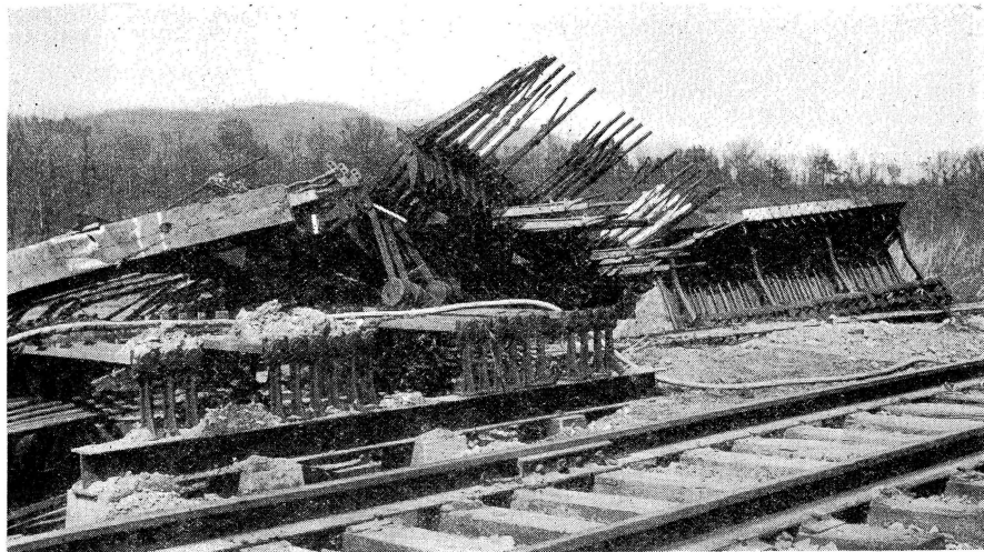
Left—The interlocking machine at Sir John's Run, Md., on the B. & O. was held by the up-and-down rods but the building floated away. Above—Demolished trunking on the Pennsylvania near Pittsburgh—wires were returned to temporary service
