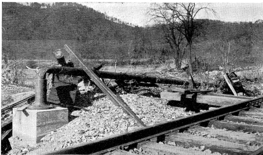
An instance on the Baltimore & Ohio where the foundation held but the signal mast bent over
