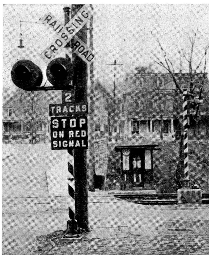
Standard A.A.R. flashing-light crossing signals are used
