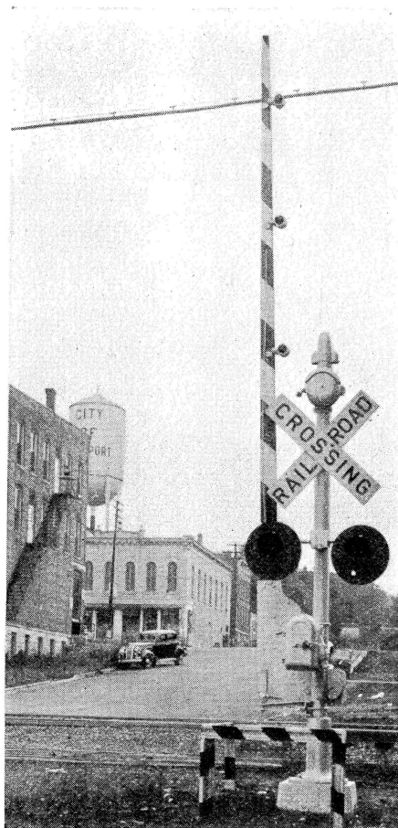
When in the raised position the gate arm is vertical
