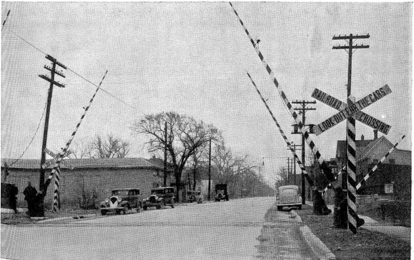
Automatic gates were installed at Fifteenth Avenue
