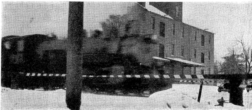
Automatic gate installation at Rochelle, Ill.
