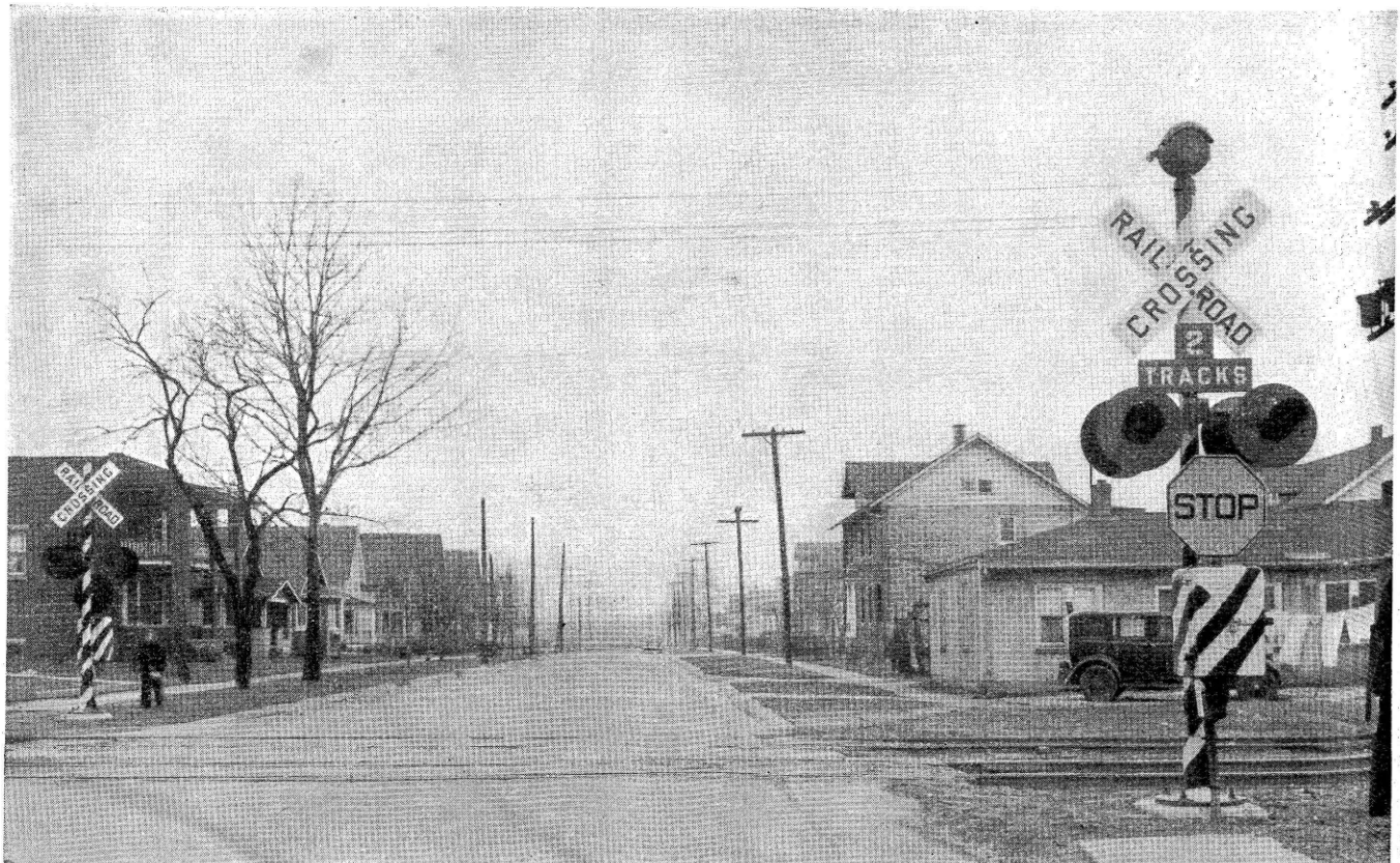
Flashing-light signal with rotating stop disk were installed at Sixteenth Avenue and Seminary Street
