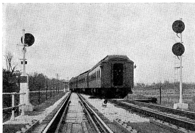
Westward home signals at West Bridge Jct. interlocking—S. P. train crossing over
