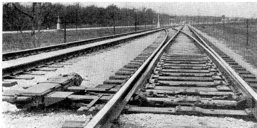
Three insulated gage plates are used in each switch layout
