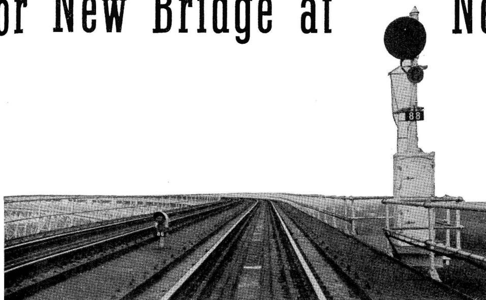
Automatic block provides for either-direction operation on both tracks
