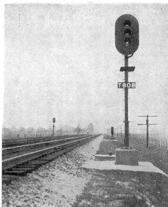
New color-light automatic block signal on the C. & O.—near Fostoria, Ohio.
