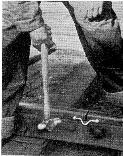
Three hammer blows will set each plug
