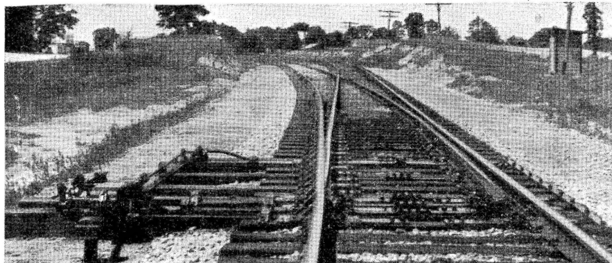
A spring switch was installed at the north end of each siding
