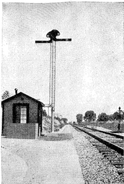
A new block office, complete with manually-operated signal, was located at the south end of each of the sidings
