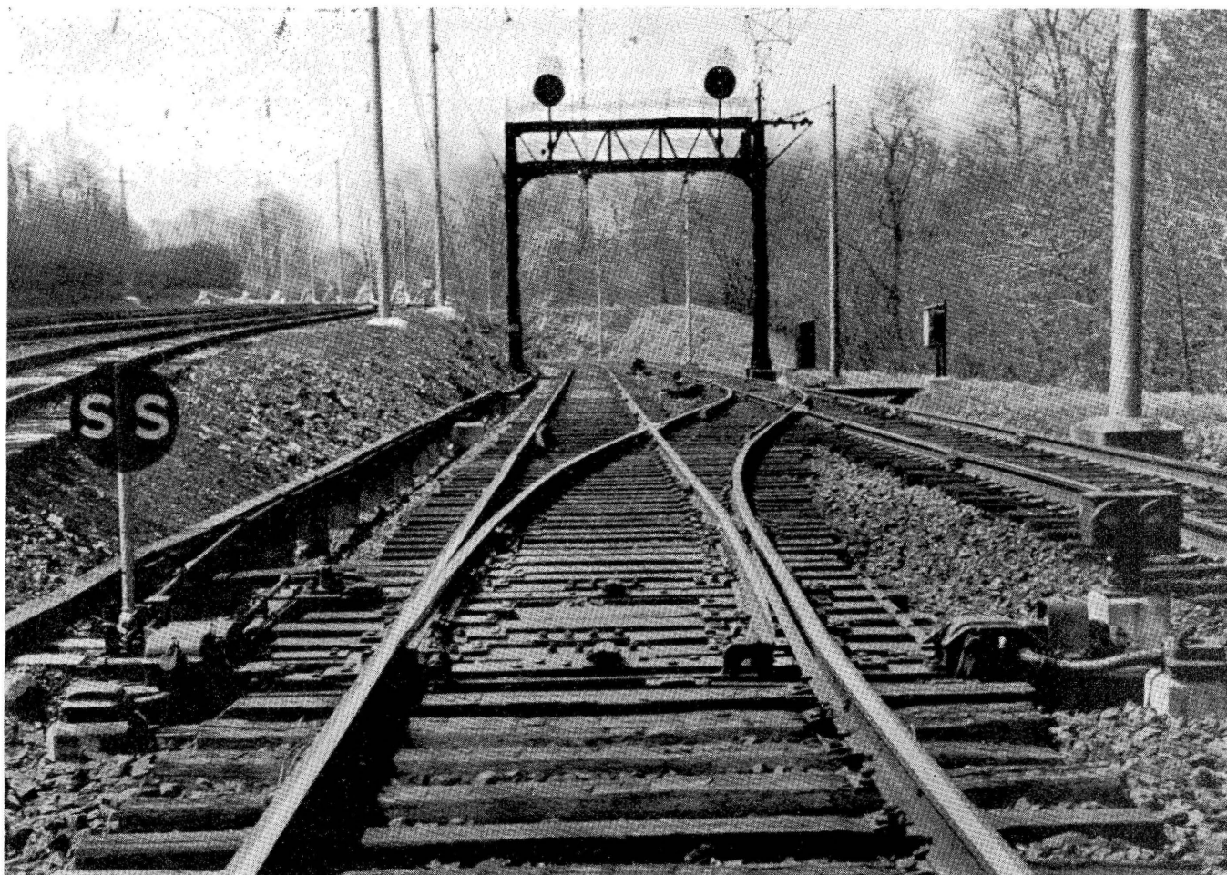
A spring switch indicator target and a color light indicator were provided
