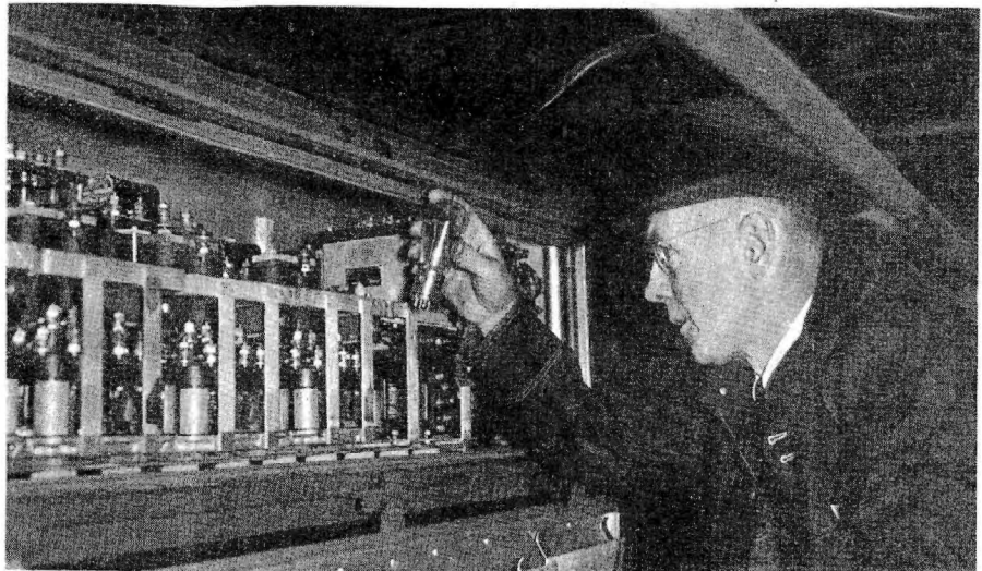
The views on this page illustrate the cab signal and train control equipment on an Interurban Electric car. Above—The amplifier, relays and decoders are mounted in a case mounted under the car
