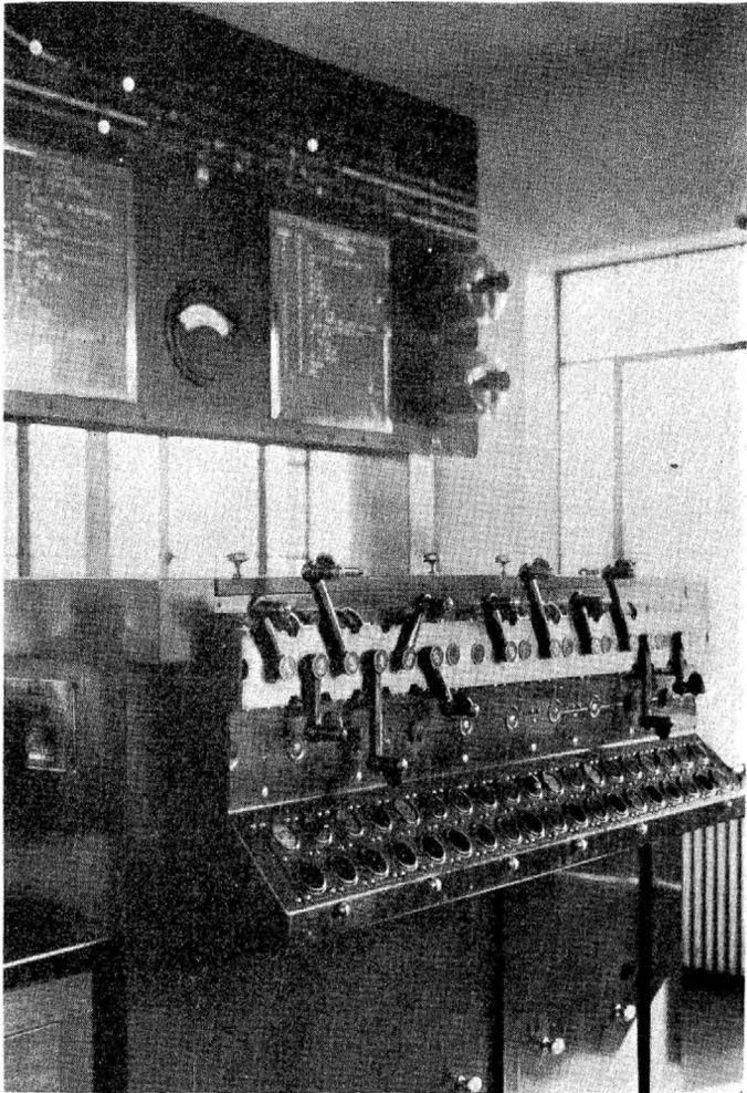
A 12-lever electric plant replaces 18-lever mechanical interlocking
