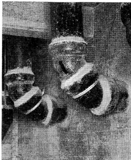
Tile duct through tower basement
