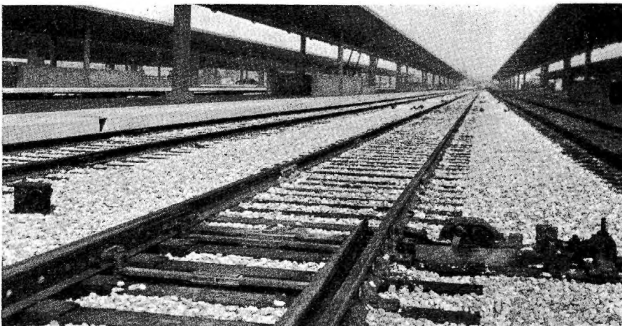
View of electric switch lamp and an oil-buffer spring switch on one of the engine-release tracks
