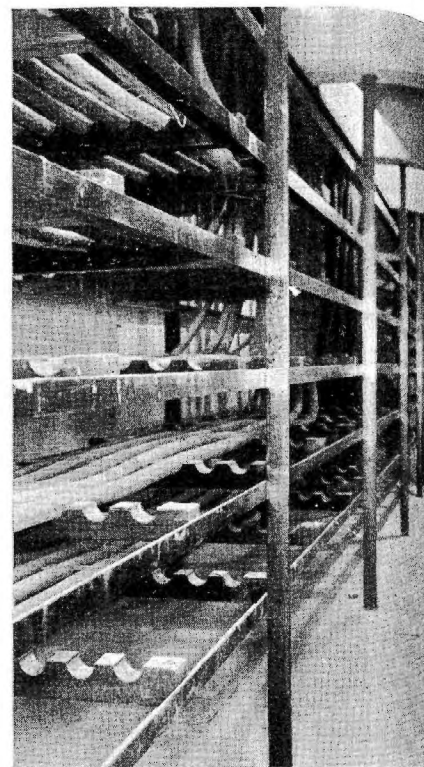
Cable rack in tower basement
