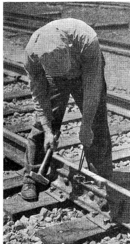
Fig. 10—A finished joint with bond being reapplied. Because of heavily beaded joint a drift hammer is used
