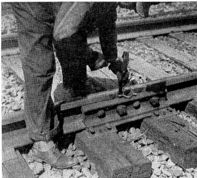
Fig. 5 Bond being removed with hammer and extractor tool
