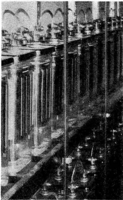
Storage cells in bungalow at North approach connection
