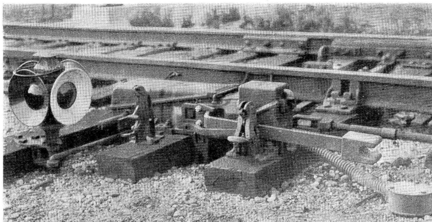
Electric switch lock 29 at Casey is controlled from the C.T.C. machine at Terre Haute
