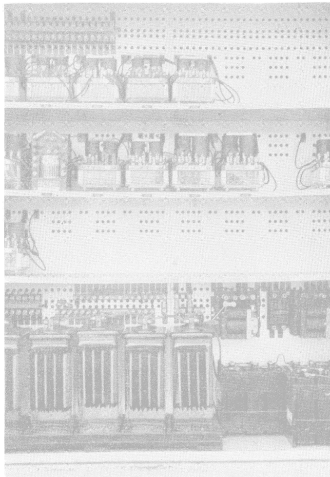
Interior view of one of the instrument cases at the crossing, showing the control relays and storage battery for control and gate operating circuits
