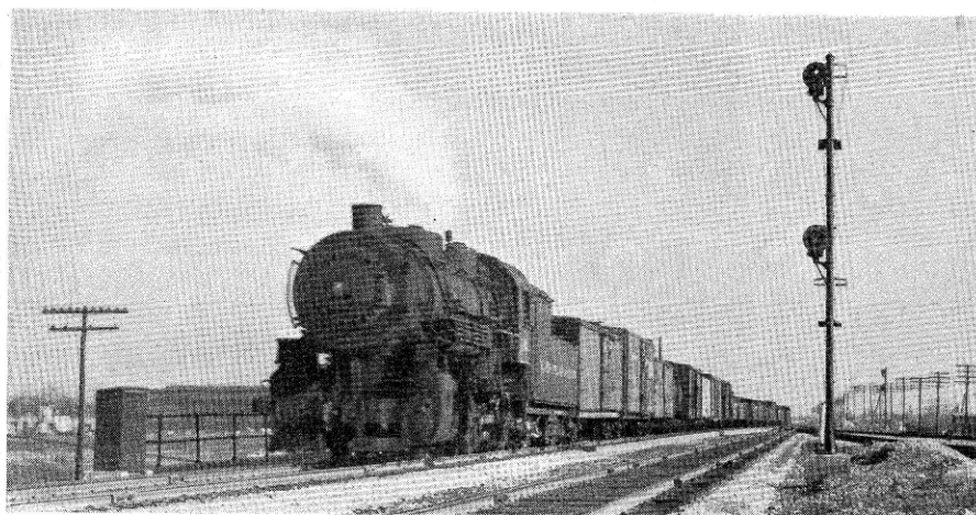
Chesapeake & Ohio freight train, bound for Clearing yard, on the Belt northward main track, showing home signal 4RAB at the west end of the new electric plant
