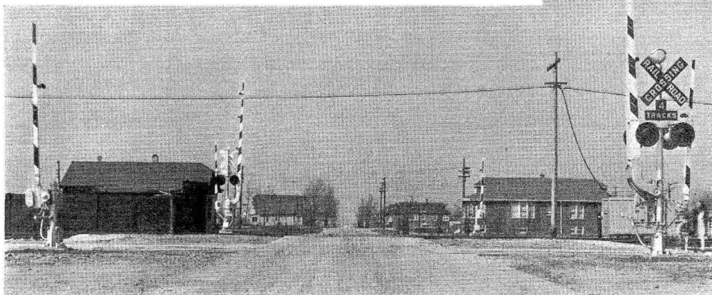
Highway crossing gates in lowered and raised positions. Note sidewalk gate at left
