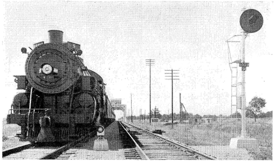
Eastbound train No. 2, the "Sunset Limited," passing over the drawbridge and by westward home signals 3 and 4. The home signals are the H-2 searchlight type
