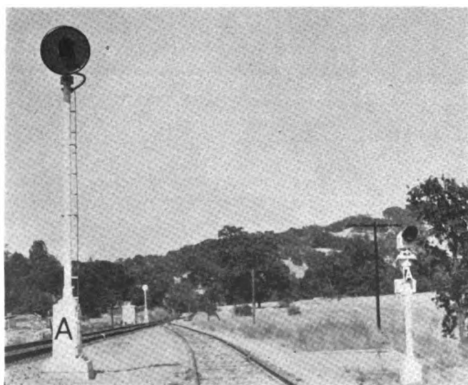
The leave-siding dwarfs are mounted on pipe masts
