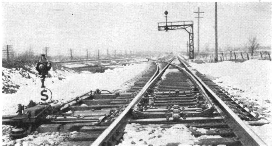
A spring switch at the east end of the siding at Leavittsburg
