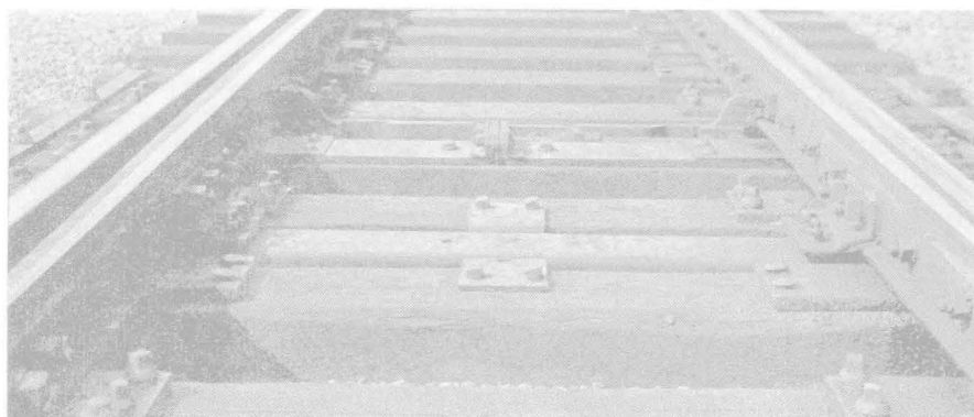
The roller bearing at the track center
