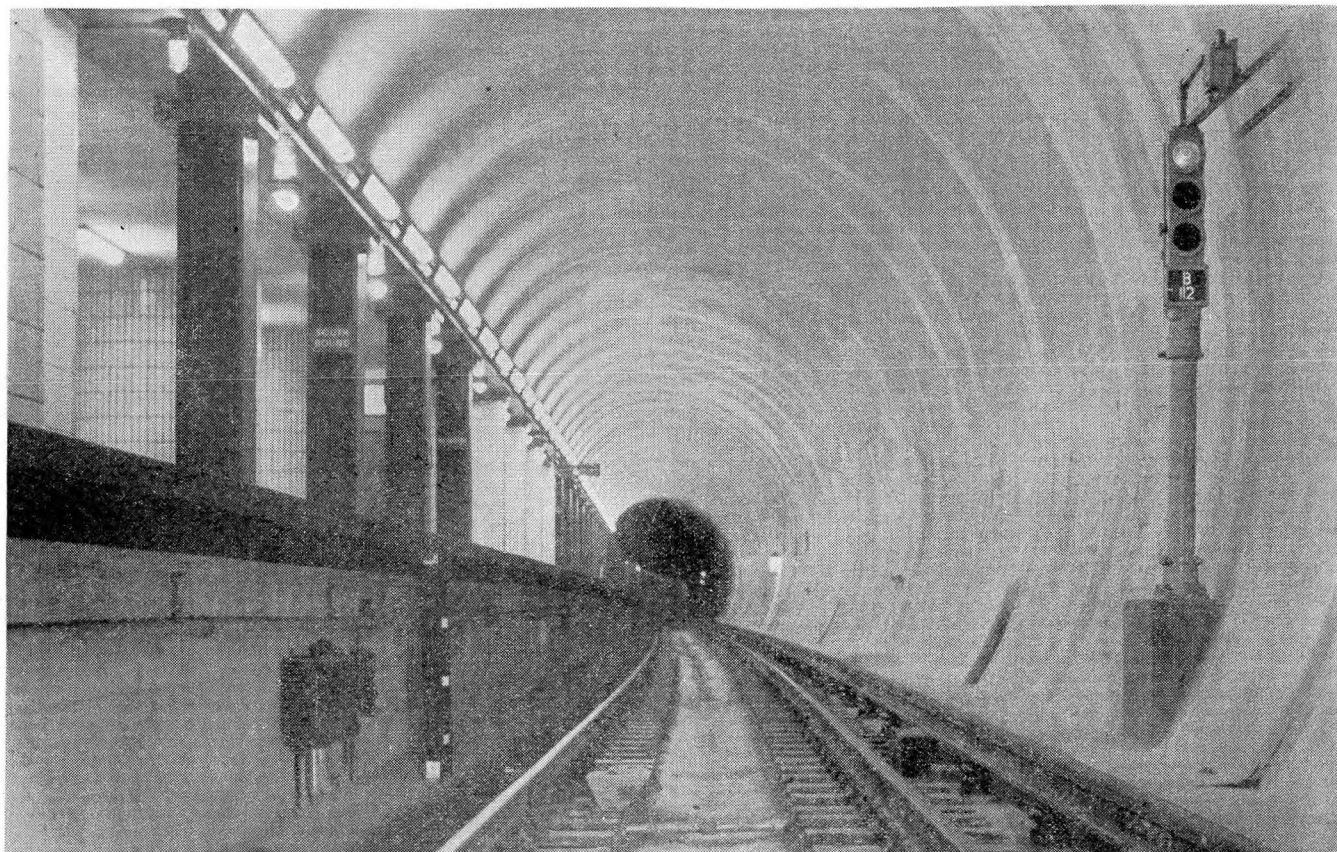
View of track along a station platform with an automatic signal at the right. Below — Motorman operating the release at an automatic signal.
