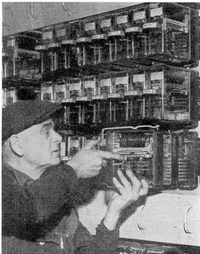
The plug-in type relays can be replaced quickly and with no wire change
