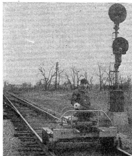
A modern one-man inspection car used by signal maintainer
