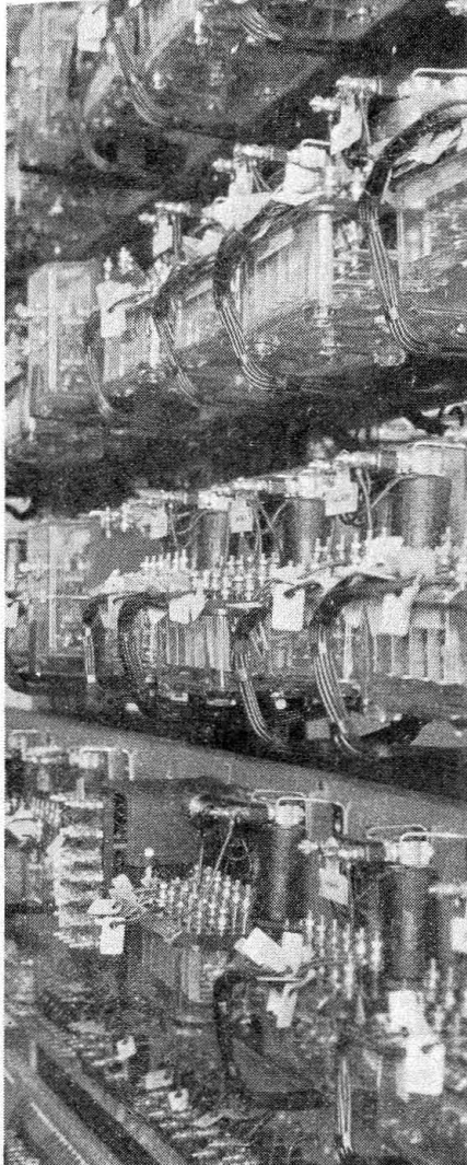
Portion of relays at Sulphur
