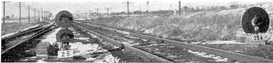
Dwarf signals 25 and 25A at Endo, showing full-size and small backgrounds
