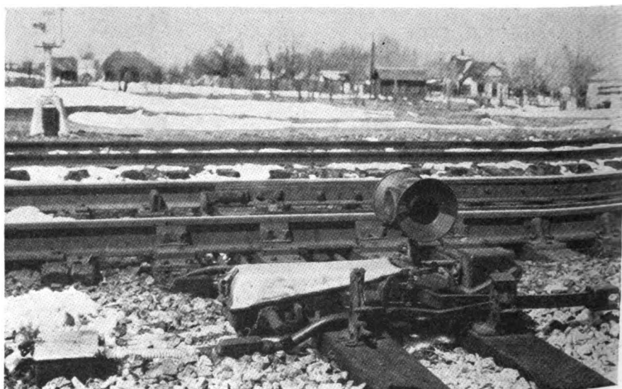
Hand-thrown switch stand with an electric lock
