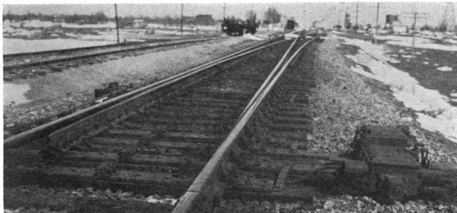
The switch layouts include heavy gage plates and adjustable braces
