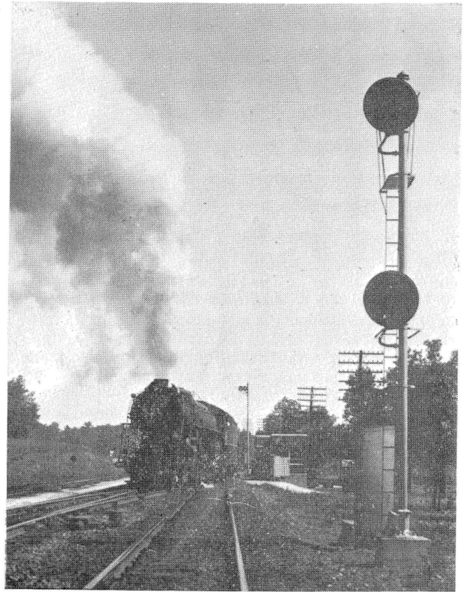
Northbound home signal at Falling Creek, showing southbound train crossing over to southbound track
