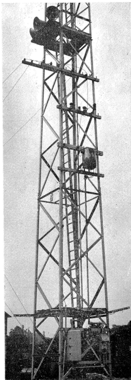
Group of three paging speakers on floodlight tower at the north end of the yard
