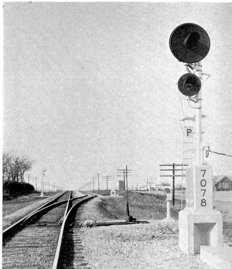
Each signal is equipped with a light-out unit which saves train stops in case of a failure of the lamp in the searchlight signal
