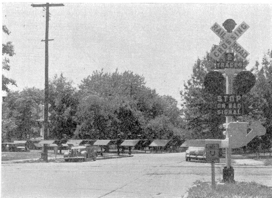
Flashers with gates lowered at the Virginia Avenue crossing. These facilities are controlled from the new interlocking plant
