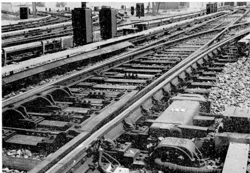
View showing electric switch machine, plates and rail braces at a switch in Pitkin yard
