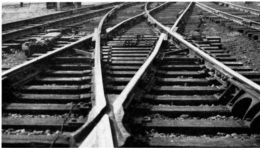
Movable-point-frog No. 24A at Bailey interlocking
