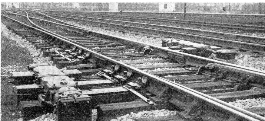
Typical electric switch machines in the new plant
