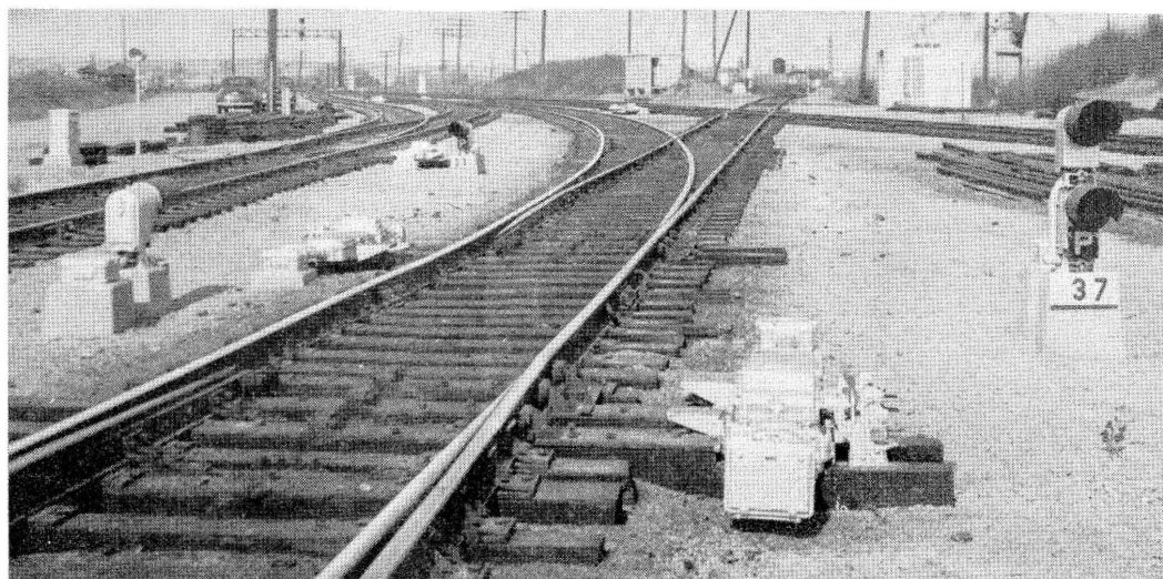
View showing switches No. 78 and No. 22 and signal No. 37
