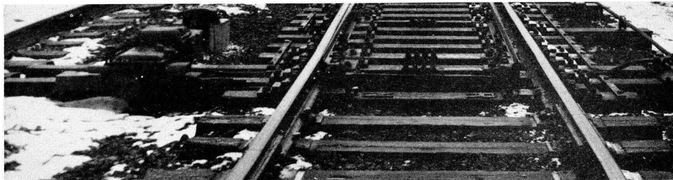
Power switch machine on crossover at Pergo
