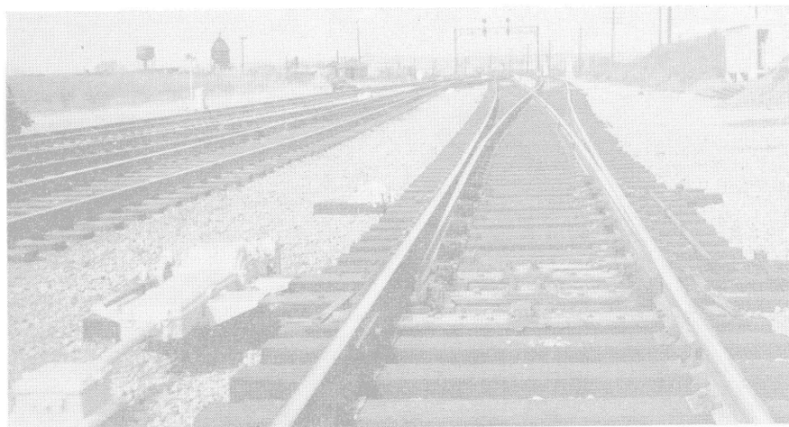
Power switch No. 68 with 33-ft. curved switch points
