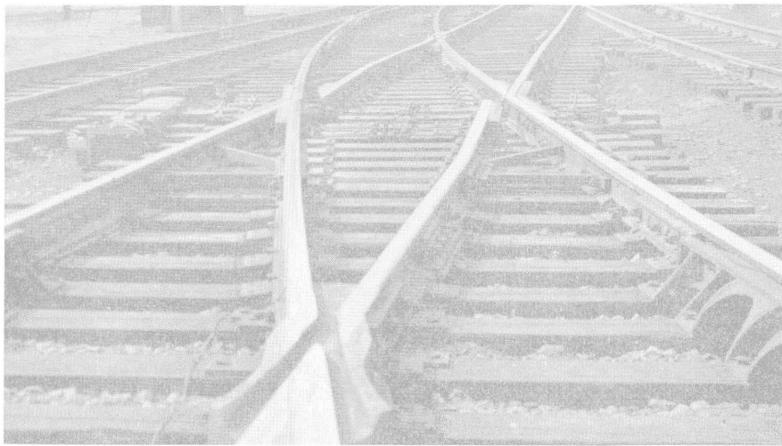
Movable-point-frog No. 24A at Bailey interlocking
