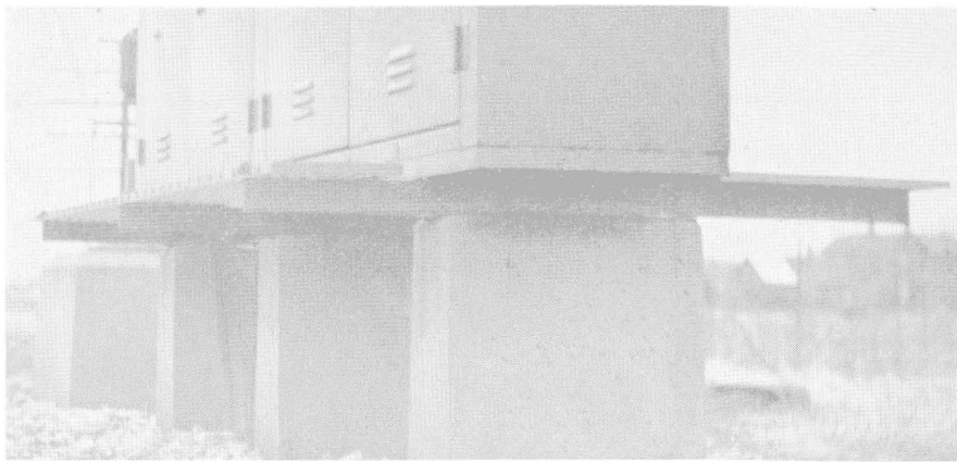
Grated-metal platforms, supported by angle irons, at instrument case on the ground
